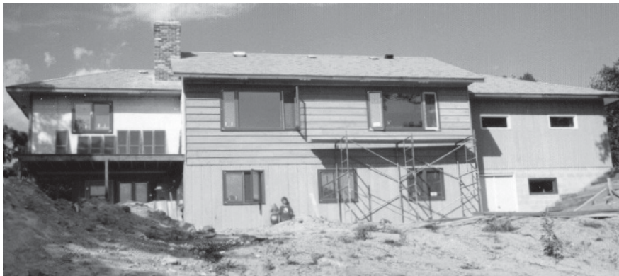
The Byron, Minnesota, house under construction.
